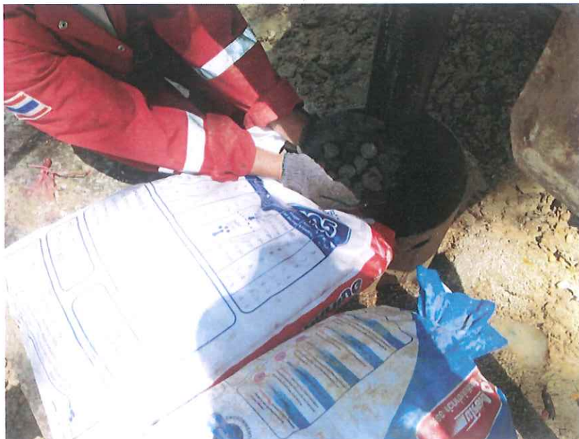
Figure 24 shows gravel pack in annulus and clay ball pack in anulus.
