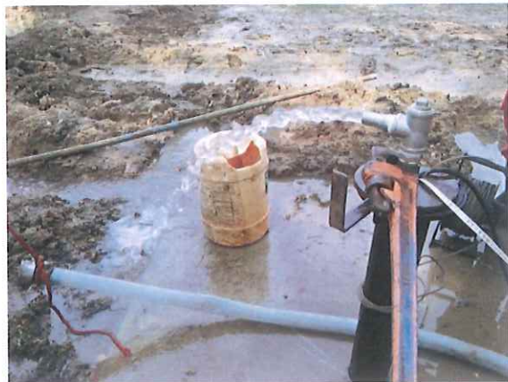
Figure 25 shows completed well and pumping test.
