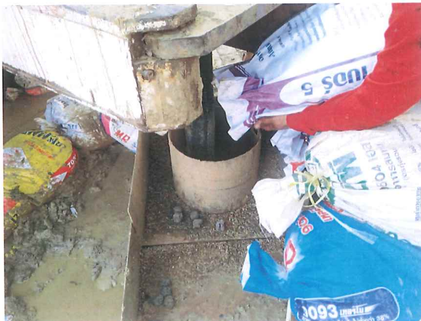
Figure 28 shows gravel pack in annulus and clay ball pack in anulus.
