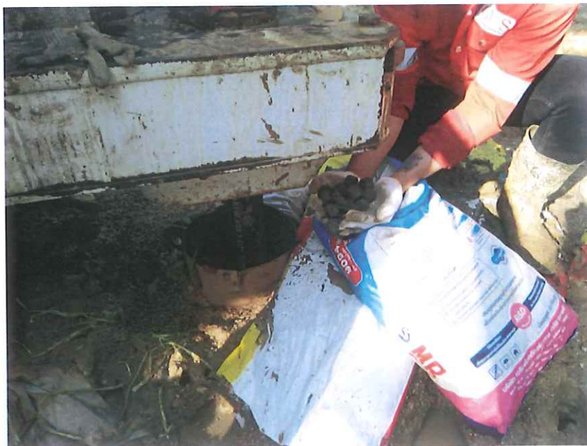
Figure 16 shows gravel pack in annulus and clay ball pack in anulus.
