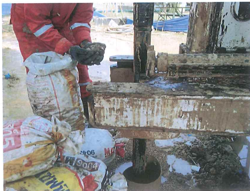
Figure 32 shows gravel pack in annulus and clay ball pack in anulus.
